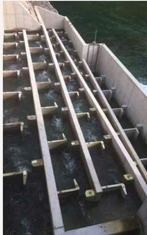
The new fishway at the at the „Große Ybbs“
